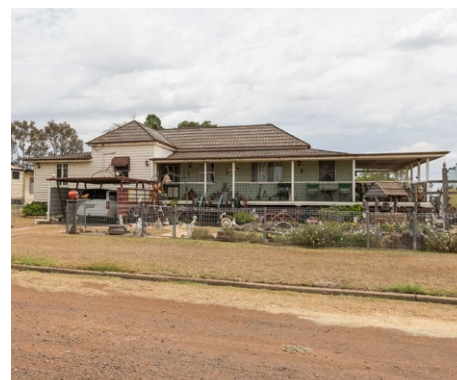
Traditional timber and tin, single storey buildings on stump footings typify Kulpi's residential character
